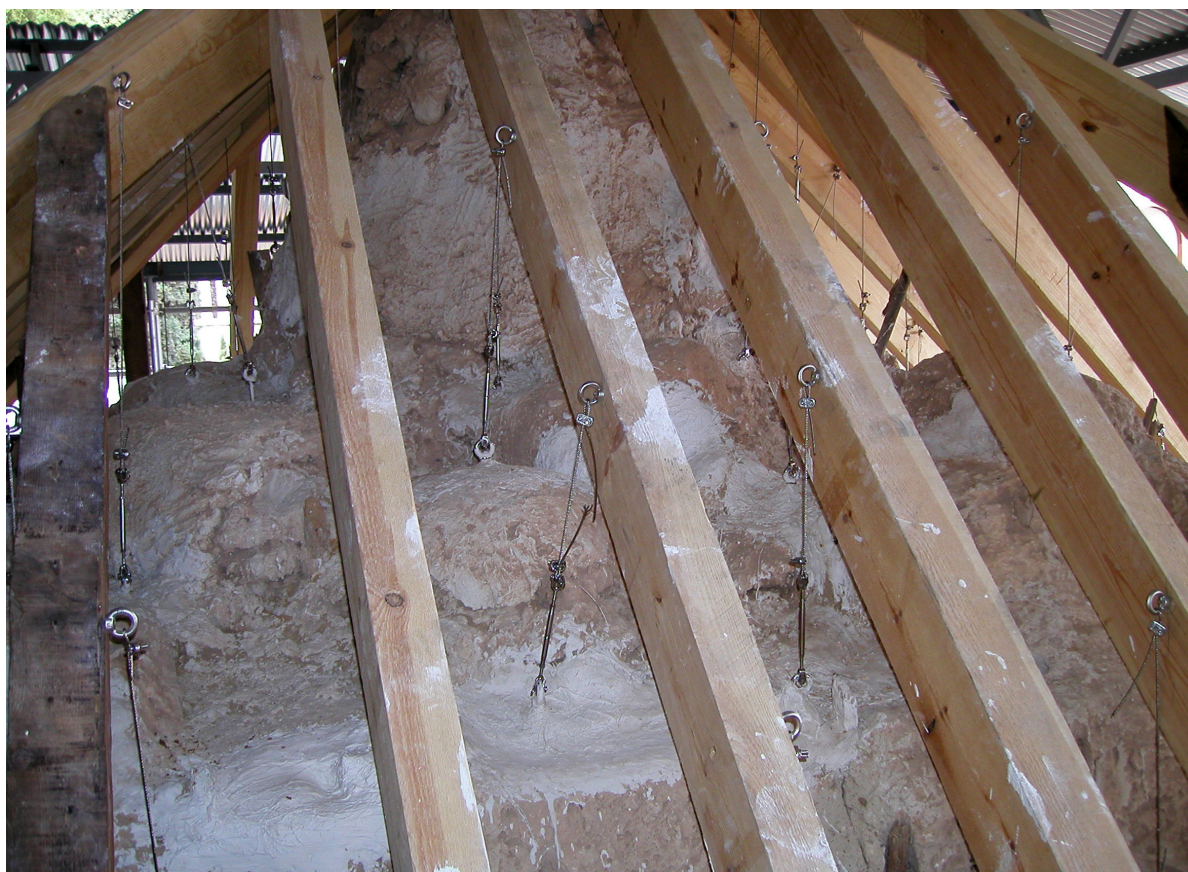
II. 16. Pedro Salmerón Escobar, 2007, photography. Tensioners placed in the new wooden framework for the elastic support of muqarnas vault M2.
