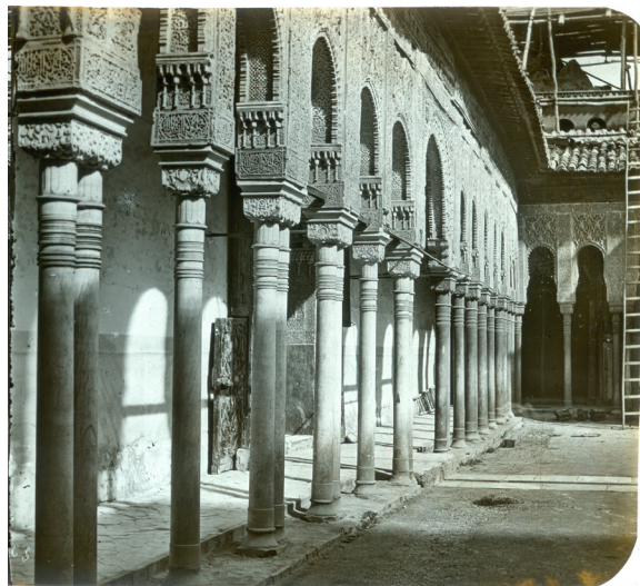
Il. 5. Soulier, 1857, photograph. Courtyard of the Lions. Carlos Sánchez Gómez Collection. The beginning of Rafael Contreras' restoration work can be seen in the background of the photograph. Once the roof was removed, the back of muqarnas vault M6 of the Hall of the Kings emerged.
