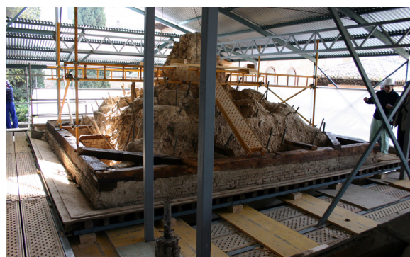
Il. 8. Pedro Salmerón Escobar, 2007, photography. View of the back of muqarnas vault M2. Restoration work protected by the cover placed over the entire area of the Hall of the Kings.
