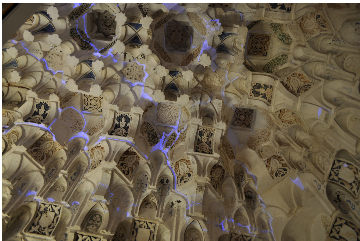
Il. 18. Photograph taken with ultraviolet light showing a detail of the final phase of restoring volume to dome 7, with work on all cracks and fissures using Alhambra plaster-based mortar.
