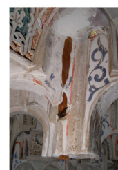
Il. 5. Location of the different wooden brace crowns which serve as support in the process of raising a dome. Their location in the photograph doesn't exactly match the topographic survey, as they weren't placed exactly perpendicular to the dome and have moved and leaned.
