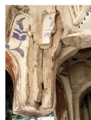
Il. 5. Location of the different wooden brace crowns which serve as support in the process of raising a dome. Their location in the photograph doesn't exactly match the topographic survey, as they weren't placed exactly perpendicular to the dome and have moved and leaned.
