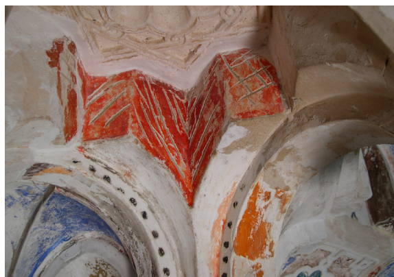
in the images below, sometimes reaches up to 7 cm. The image above shows large forged angled nails (in blue), which were introduced in later 19th century works to guarantee its stability and prevent it from collapsing.
