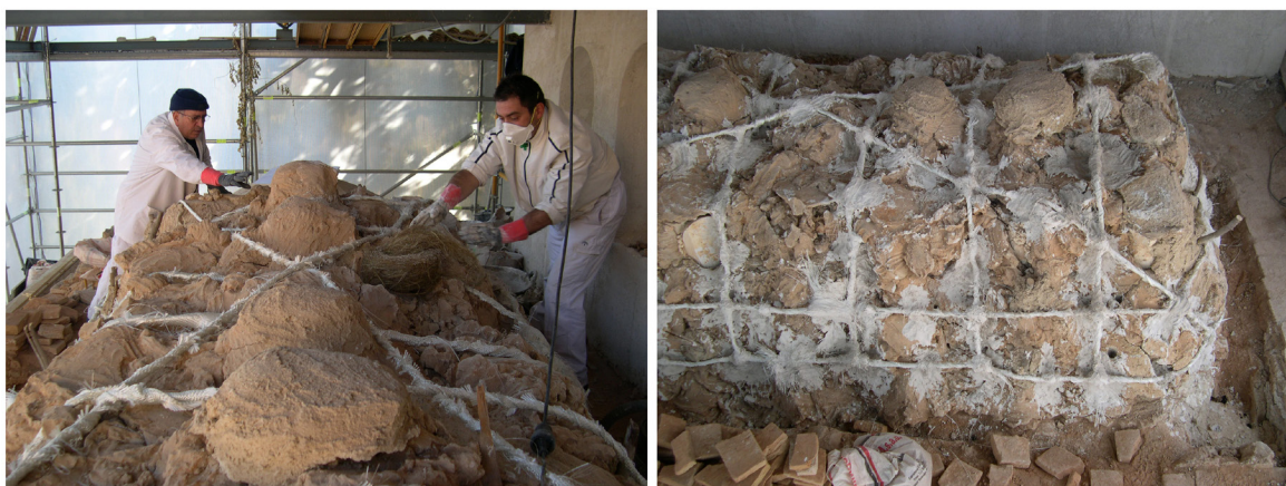
Il. 15. Restoration process that involved placing a fibreglass mesh fixed with esparto grass mixed with plaster on the back of dome 7.
