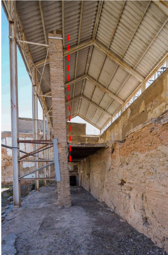
IL. 14. Pepe Marín. Loss of verticality in the south portico pillars (2016). APAG.
