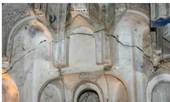
Il. 10. Pedro Salmerón Escobar, 2007, photography. Cracking typical to the accumulated deterioration of the muqarnas vaults.
