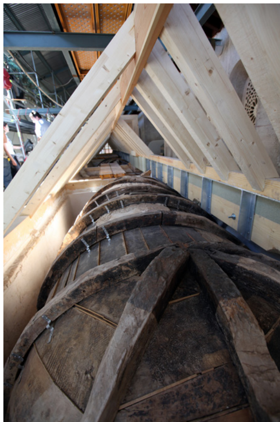
Il. 23. Pedro Salmerón Escobar, 2010, photography. New wooden roof frame over the painted wooden vaults. Vault B3 in the foreground where the ribs and curved and assembled boards can be seen.
