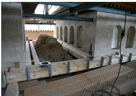
Il. 21. Pedro Salmerón Escobar, 2010, photography. Double glued laminated timber beam supporting the main channel and the structure. Positioning of PVC drains. The back of muqarnas vault M5 can be seen between the main pavilions M4 and M6.
