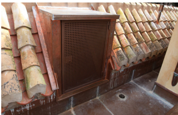
Il. 22. Pedro Salmerón Escobar, 2011, photography. Copper plate finishes on main channels and embrasure for access to roof for maintenance. A static Hoover in sheet copper can be seen in the background.
