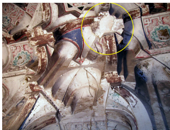
Il. 11. Pedro Salmerón Escobar, 2007, photography. Cracks in the muqarnas vaults and a spreading perforation towards the interior due to the fasteners installed in 1857 (marked with a yellow circle).
