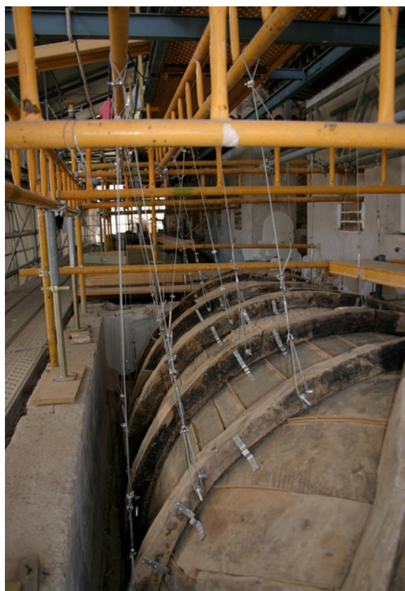
Il. 27. Pedro Salmerón Escobar, 2009, photography. View of the suspension system used in vault B3 using auxiliary scaffolding.
