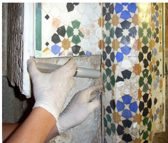
II. 8. © Ártico. Layer fixation. Report on the conservation and restoration work on the plinth of the Sala de los Reyes, Alhambra (Granada), 2011-2012.
