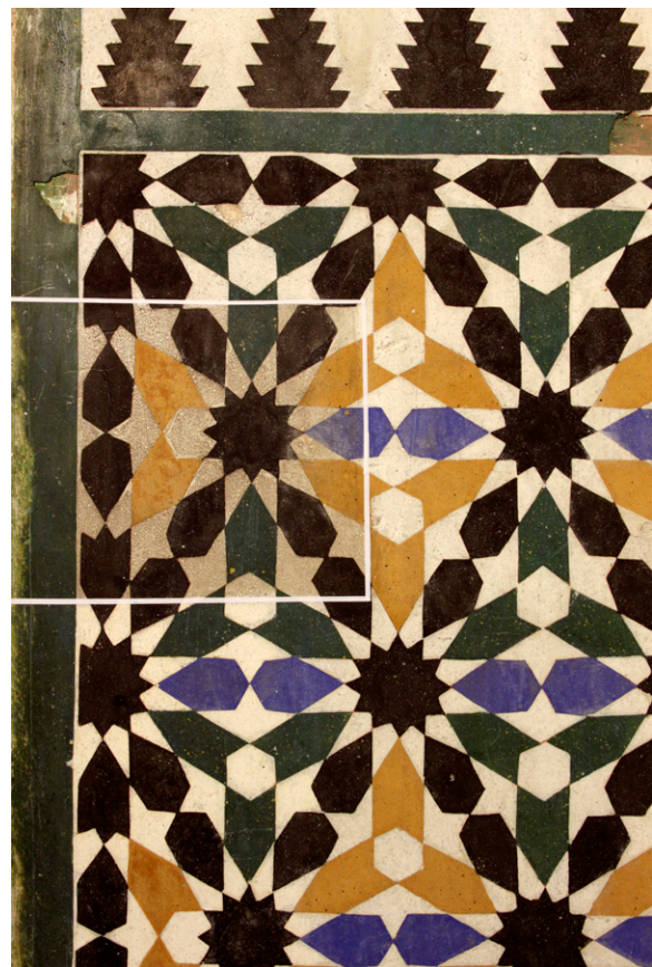
II. 10. © Ártico. Cleanliness indicator. Report on the conservation and restoration work on the plinth of the Sala de los Reyes. Alhambra (Granada). 2011-2012.
