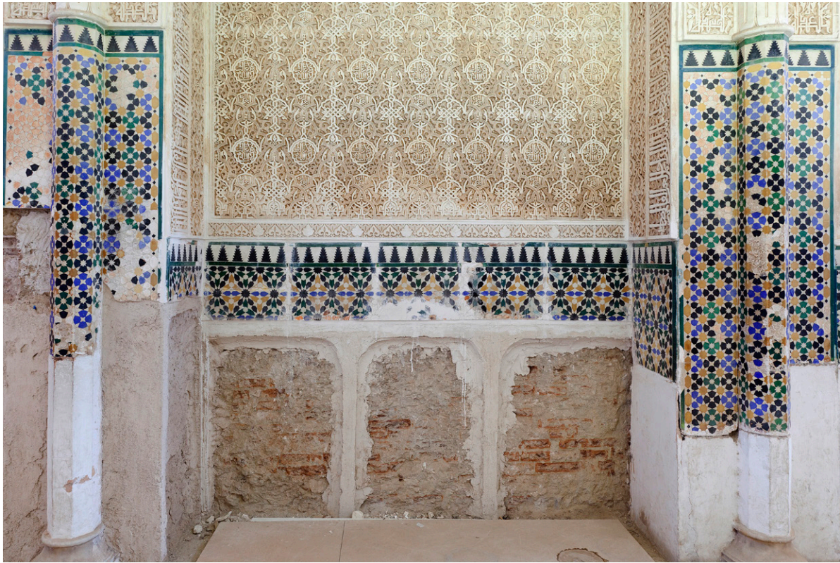
II. 6. © Ártico. Preparation and restoration of the walls. Report on the conservation and restoration work on the plinth of the Sala de los Reyes. Alhambra (Granada). 2011-2012
