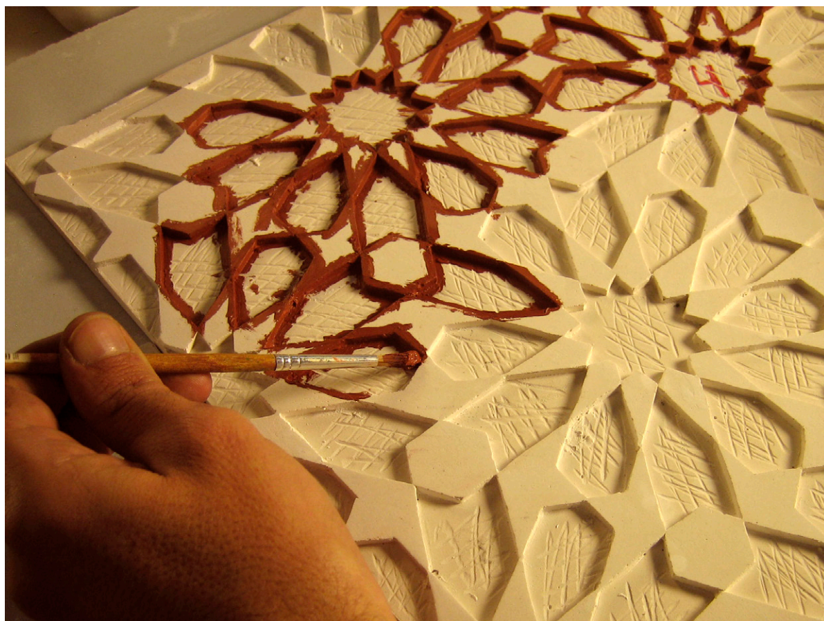
II. 13. © Ártico. Priming of the positive. Report on the conservation and restoration work on the plinth of the Sala de los Reyes. Alhambra (Granada). 2011-2012.
