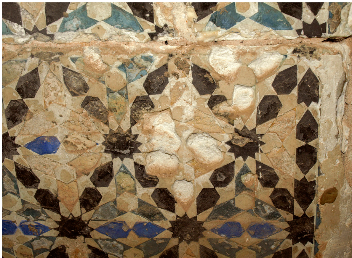
II. 5. © Ártico. Degradation caused by damp on a panel with a stucco reproduction by Rafael Contreras. Report on the conservation and restoration work on the plinth of the Sala de los Reyes. Alhambra (Granada). 2011-2012.
