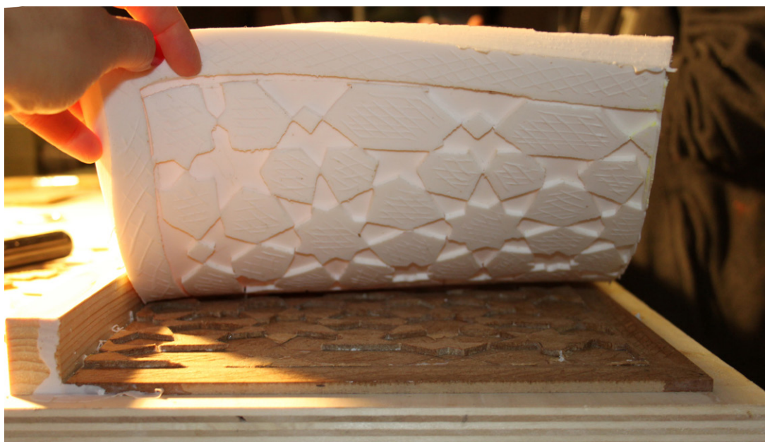
II. 12. © Ártico. Mould. Report on the conservation and restoration work on the plinth of the Sala de los Reyes. Alhambra (Granada). 2011-2012.
